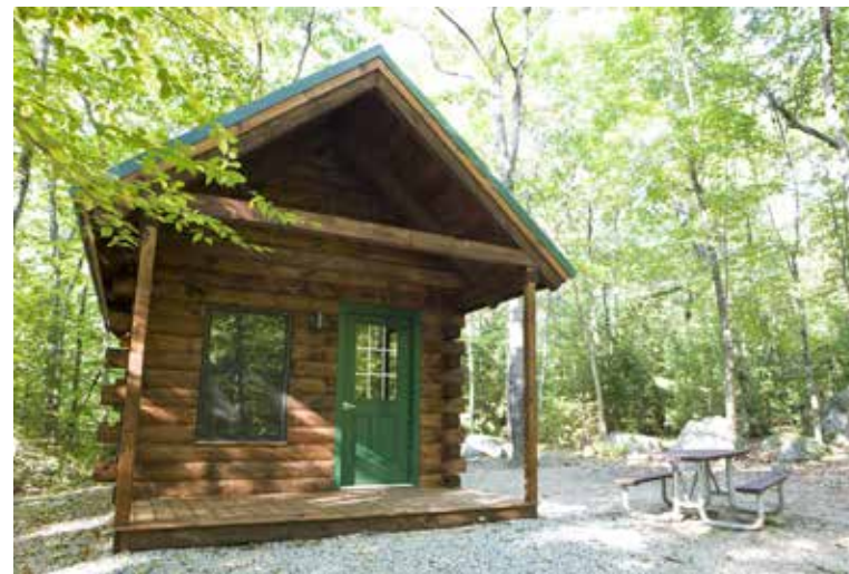
PAWTUCKAWAYS RECENTLY BUILT CABINS
