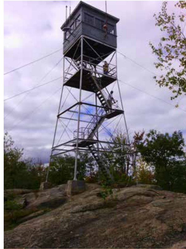
PAWTUCKAWAY STATE PARK FIRETOWER
